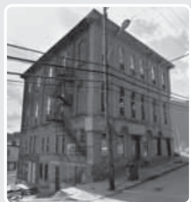
At the corner of Steuben and Wabash streets sits the former home of Saint Clair Lodge #362
