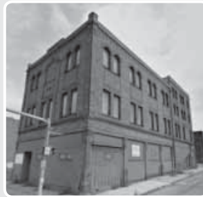
Hall of Hazel Glen Lodge #1043 – Notice the three links front & center of the building
